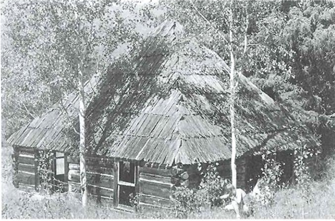
The roof of the Ray farm house was modelled on the traditional kekuli, or pit house, of B.C.'s interior native peoples. (TG)
